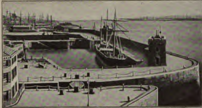
Clarence Dock, Liverpool. The rise and fall of the tides in the river Mersey is so great that immense stone docks have been built, into which the ships pass at high tide through gates like the gates of a canal. The gates are then closed, and the water level in the dock remains the same. Passengers are landed at a floating stage.
